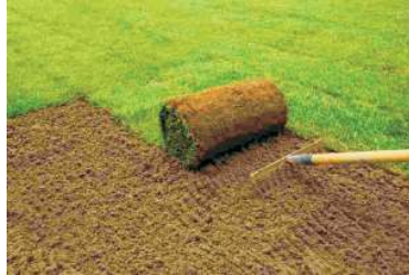
Lawn Grass Installation
