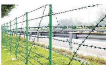
Barbed Wire Fencing
